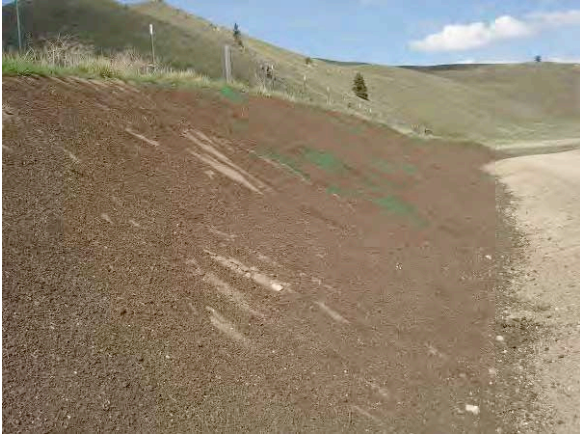
Figure A-11. Compost/seed applied on a road slope
