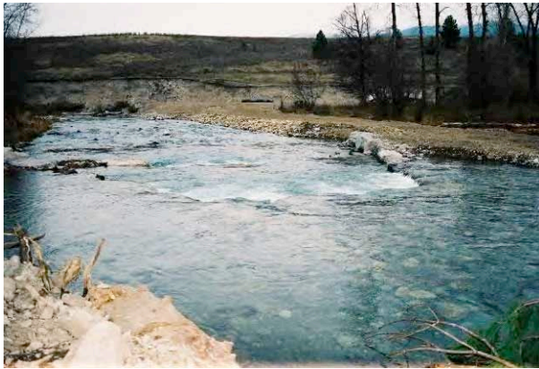
Figure A-5. Cross Vane.
