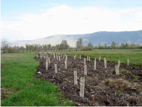
Figure A-6. Secondary irrigation canal immediately after complete ditch plugging, microtopography enhancement and revegetation techniques were implemented.
