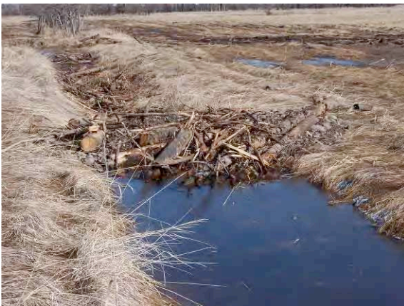
Figure A-7. Secondary irrigation canal immediately after partial ditch plugging to enhance adjacent wetland hydrology was implemented.
