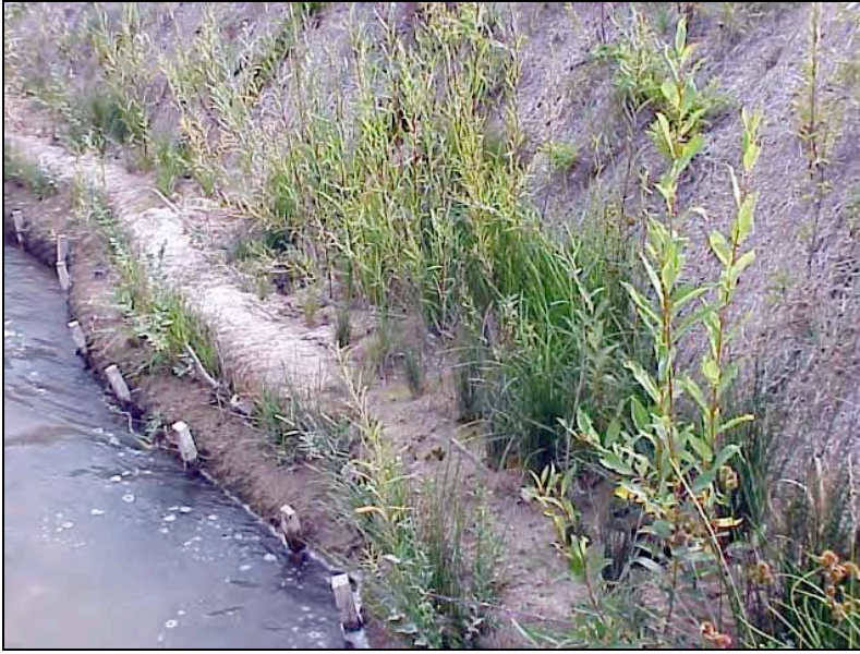
Figure A-30. Coir log used to stabilize the toe of streambank.
