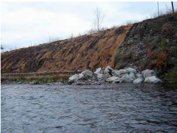
Figure A-10. Coir erosion blanket along the Jocko River near Arlee.
