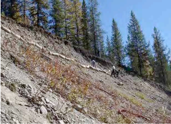
Figure A-12. Example contour wattle installed on contour to reduce slope length and control slope erosion.
