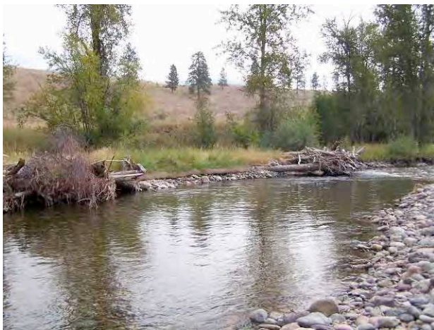
Figure A-1. Constructed woody debris jam.
