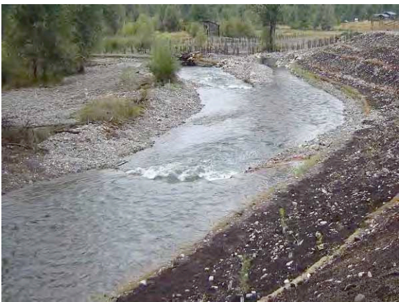
Figure A-4. J-Hook vane.
