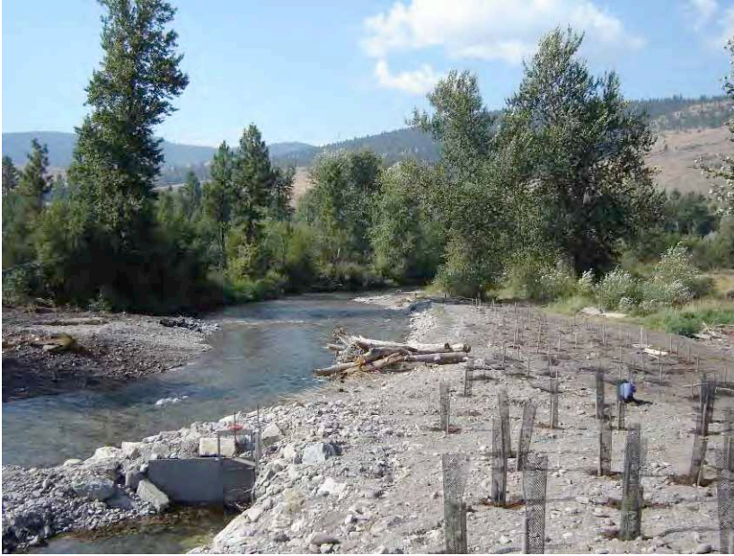
Figure A-23. Bankfull benches facilitate the reestablishment of the herbaceous and woody plant community in the near-bank zone.
