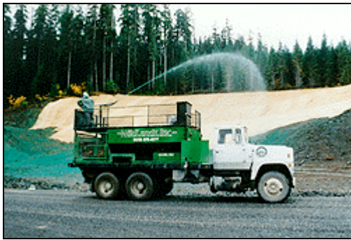
Figure A-20. Hydroseeding.
