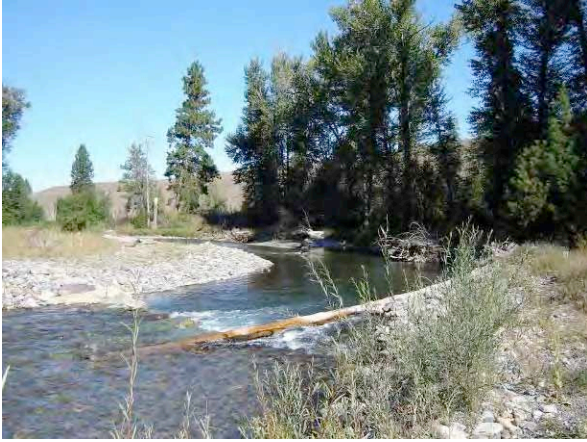
Figure A-3. Log straight vane.
