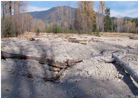
Figure A-16. Constructed microtopography as part of new floodplain construction.
