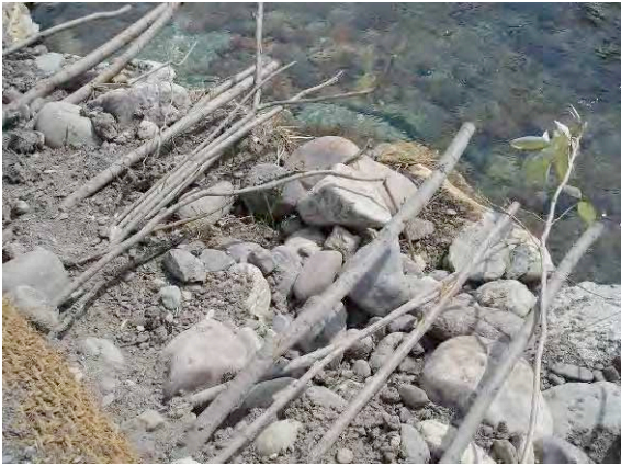
Figure A-21. Live willow cuttings installed between soil lift layers
